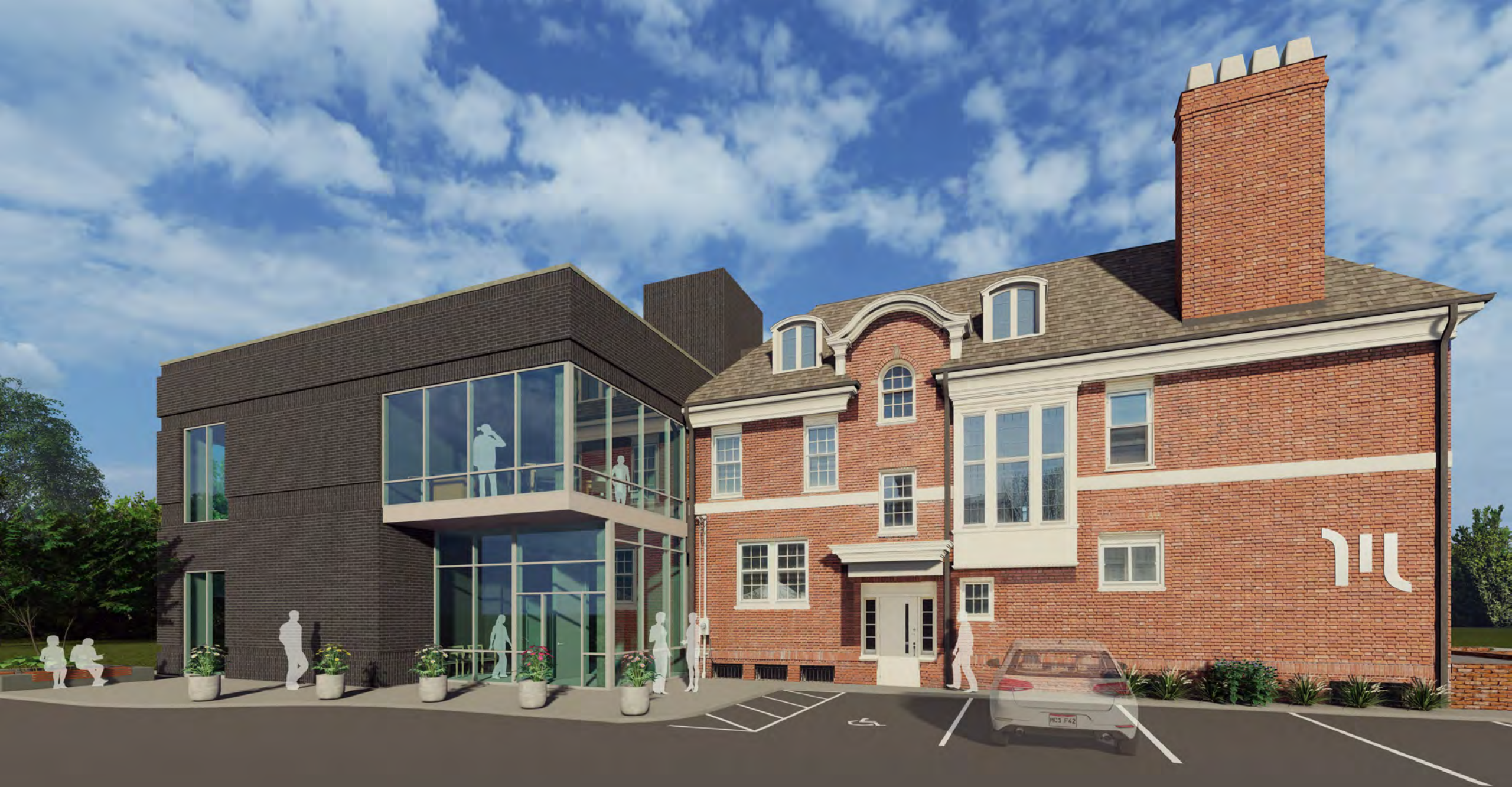
View from South of new Entry
